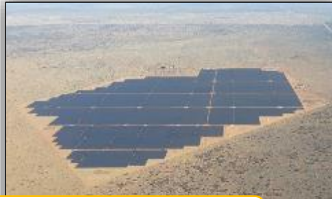
Adams 82.5 MW PV
